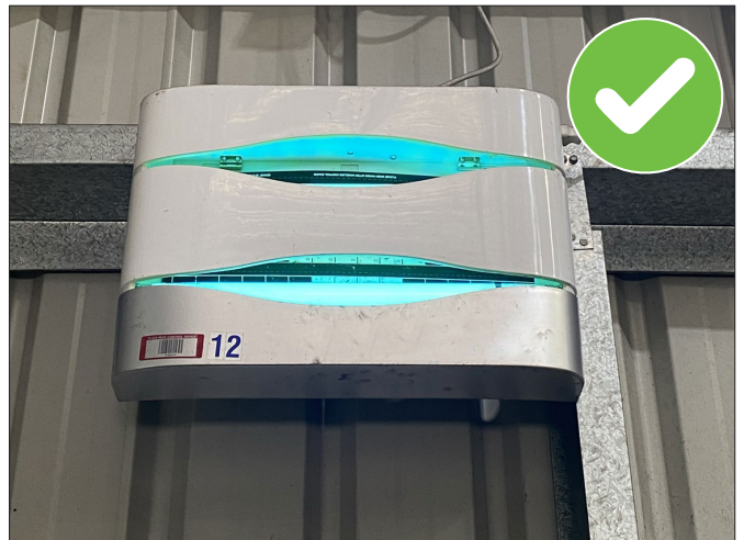
Image C9:8 | Good practice example of ultraviolet light used to attract flying insects, which are then captured on glue boards instead of being electrocuted. These are widely used in packing sheds and protected cropping environments due to their low risk of insect fragmentation (unlike electric zappers).
