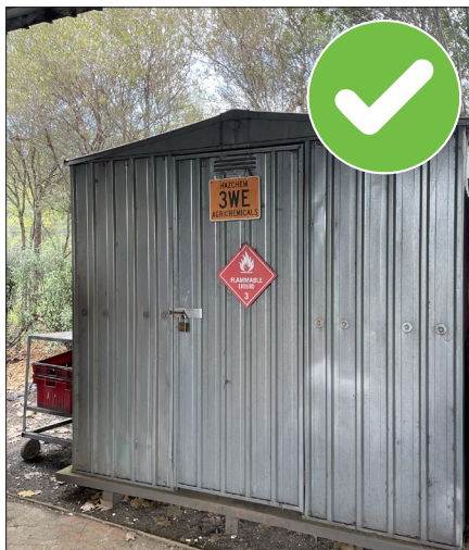
Image C8:4 | The chemical store should be structurally sound, secure, adequately lit, well ventilated, constructed to protect chemicals from direct sunlight and weather exposure.
