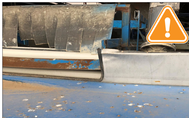
Image C10.4 | Unacceptable practice example of a packing line with rust and flaking paint which can introduce a potential hazard.
