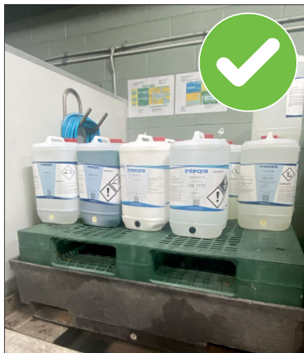
Image C8:3 | Chemicals should be stored within the original containers, adequately labelled and kept in a designated storage area.
