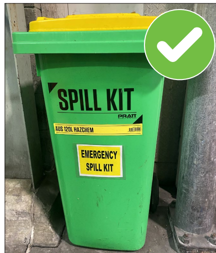
Image C8:5 | The chemical store should be equipped with a spill kit to contain and manage chemical spills
