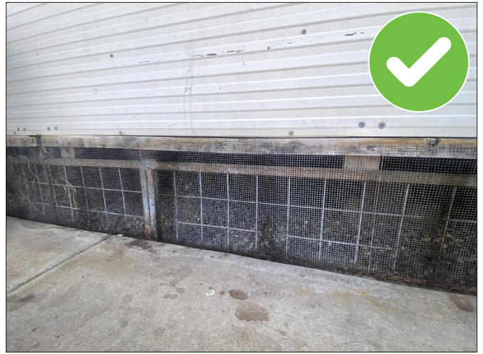
Image C9:6 | Good practice example of under-building mesh, providing protection from pests.
