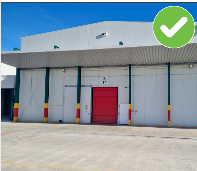
Image C9:1 | Good practice example of a tidy and clean area outside a facility.
