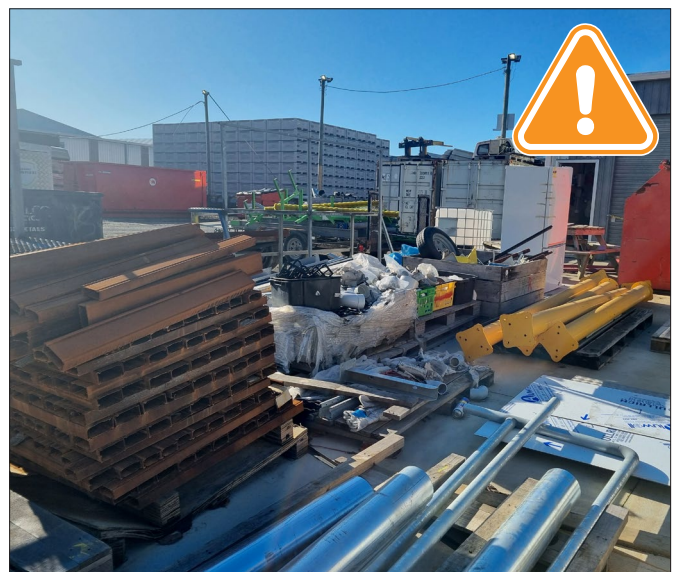
Image C9:2 | Unacceptable practice example with external areas that are not adequately maintained, creating conditions that may harbour pests and increase risk of contamination.
