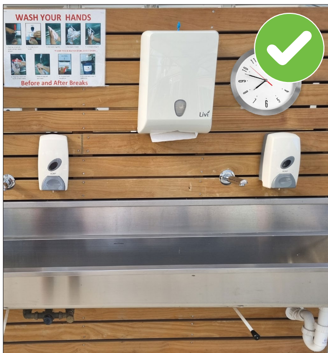
Image C14:2 | Handwashing stations should be clean, clearly signed and stocked with soap and single-use paper towels. A visible 20-second timer should be provided to support effective hand hygiene. Any glass or hard plastic items used for timing should be recorded in the glass and hard plastic register.
